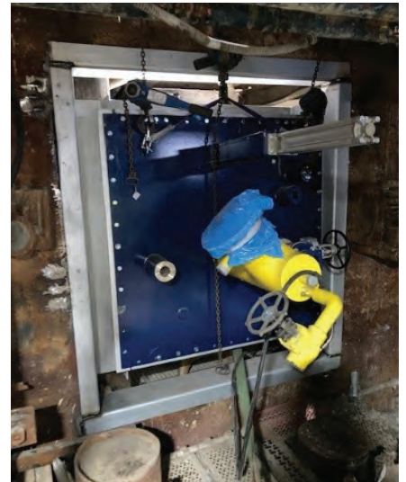
New burner being installed (Photo: RJM International)
